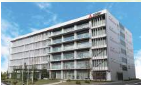
Air-Conditioning & Refrigeration Systems Works
